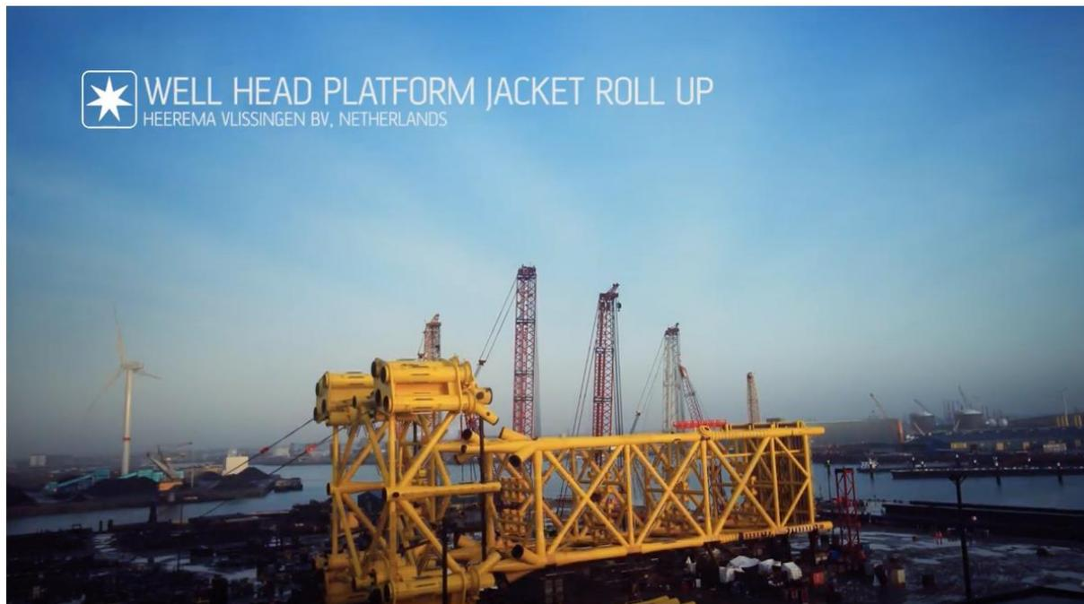
Figure 3: Production phase of the jacket construction in the Netherlands– The right part is being twisted 45 degrees , so the parts fit and can be welded together.
