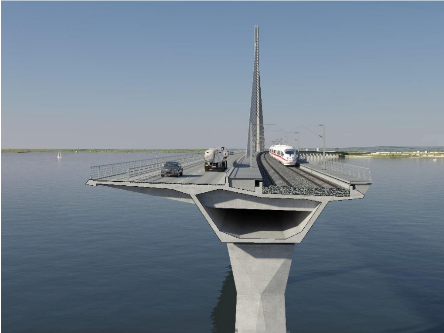
Figure 2 - Cross section of the bridge superstructure. (Note that the rail tracks post this rendering were changed to a slab-track solution, as opposed to the shown ballasted solution.)
