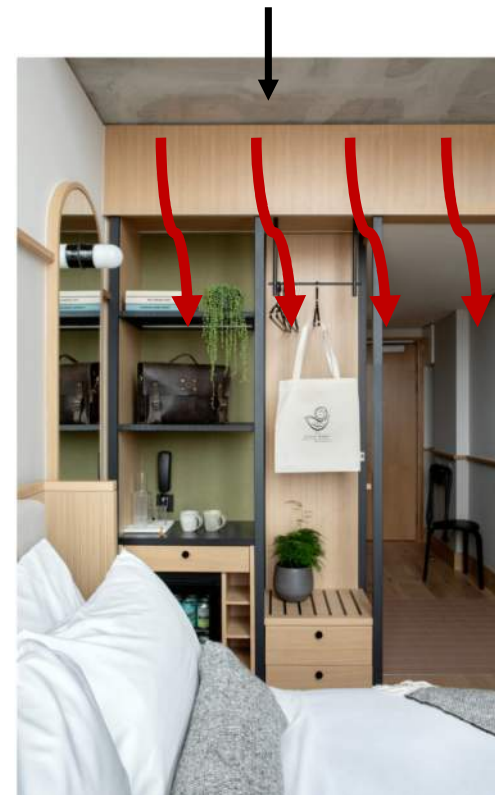
Exposed slab releases heat at night
