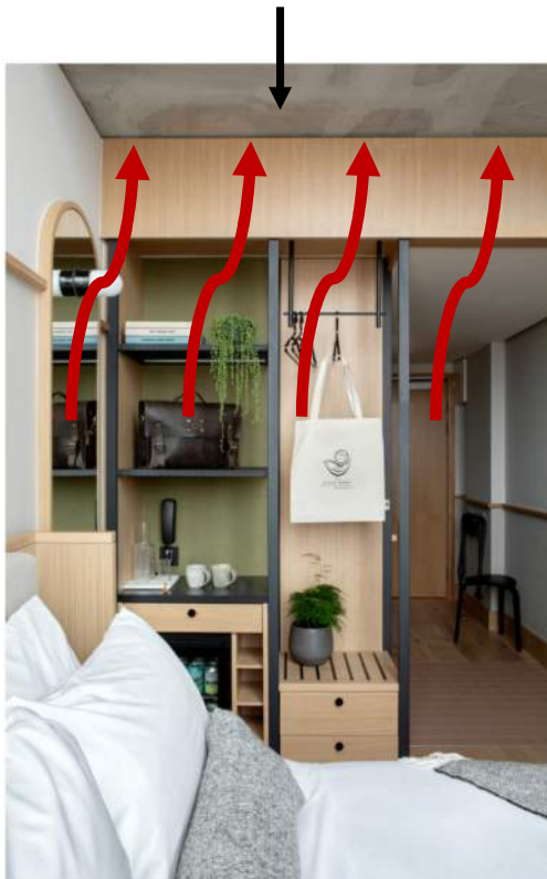
Exposed slab absorbs solar gain during the day
